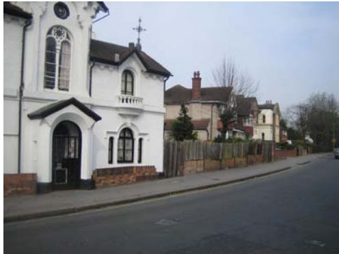
Picture 4.21 Locally Listed building with character on Lancaster Road
