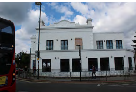
104. Former public house on Portland Road, Portmanor, now known as The Signal
