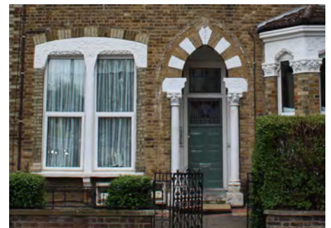
84.Decorated door and window surrounds, and arched opening and stone dressings. Ironwork railings and gate still in place.
