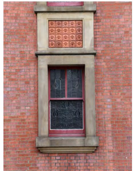
92. Red brick with stone and tile details, with sash window and stained glass (Stanley Halls)
