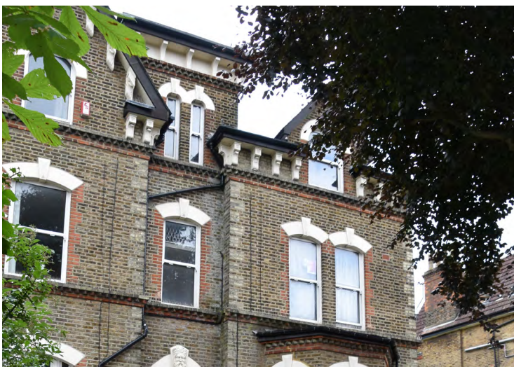
65. Example of London stock brick, red brick and stucco detailing on Warminster Road
