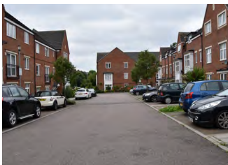
14.Recent residential development on Chalfont Road
