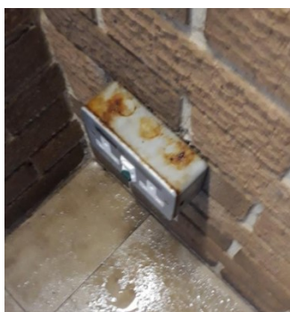
< Condense dropping on outlets not IP rated.
