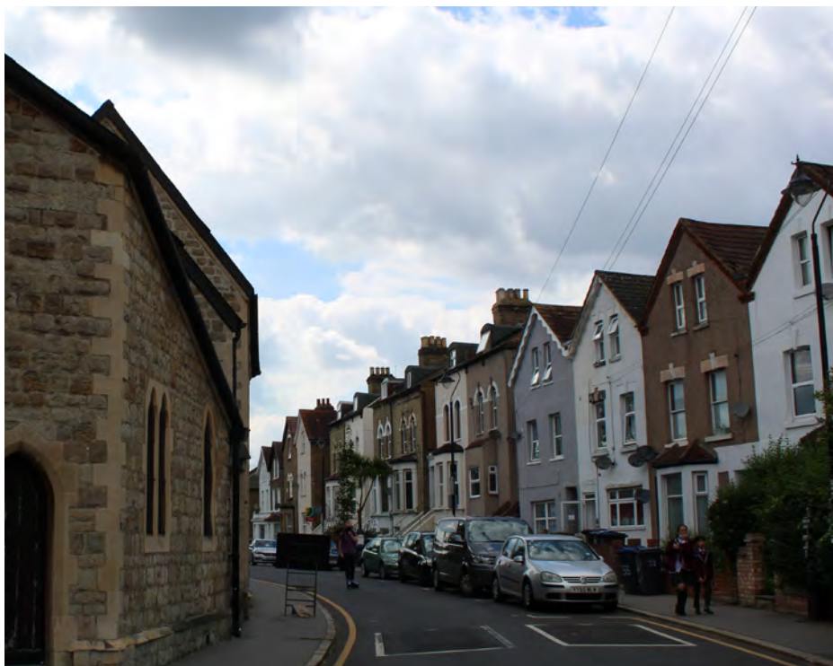
131. View west along Albert Road
