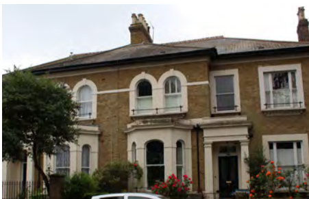
86. London stock brick, stucco, and slate roofing
