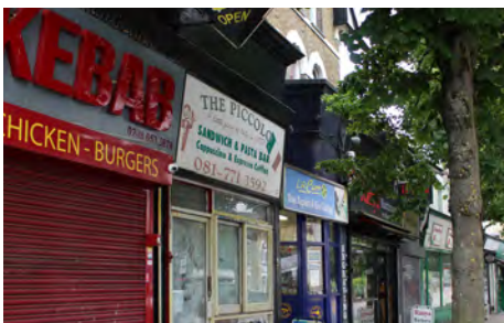
87. London stock brick and some timber shopfront detailing surviving
