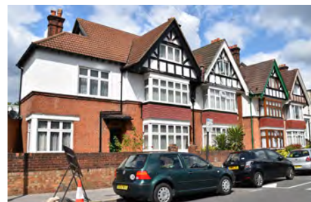
11. Semi-detached houses on Albert Road
