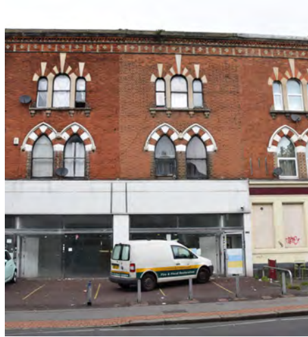
148. Example of a vacant building within the Conservation Area
