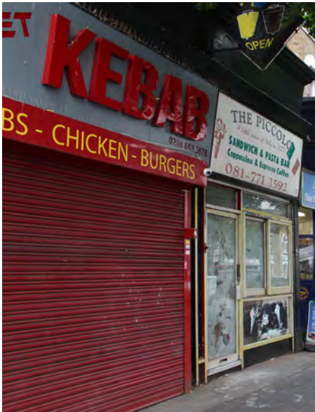
143. Example of the effect of shutters on the streetscape
