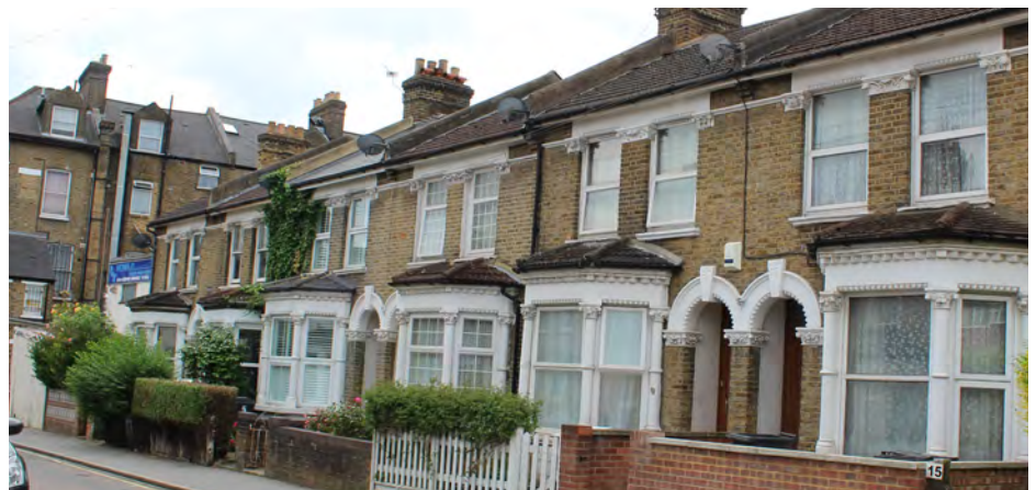
43. Consistent form, scale, height and mass of residential buildings on St Dunstan's Road
