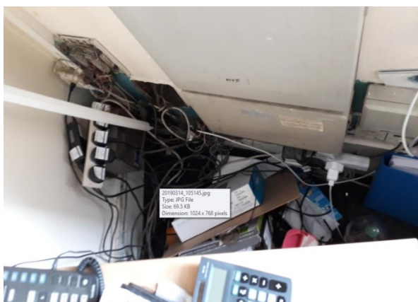
< Condense dropping on outlets not IP rated.
