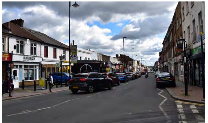
52. South along Portland Road
