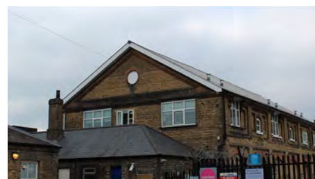
8. The goods shed at Norwood Junction Station
